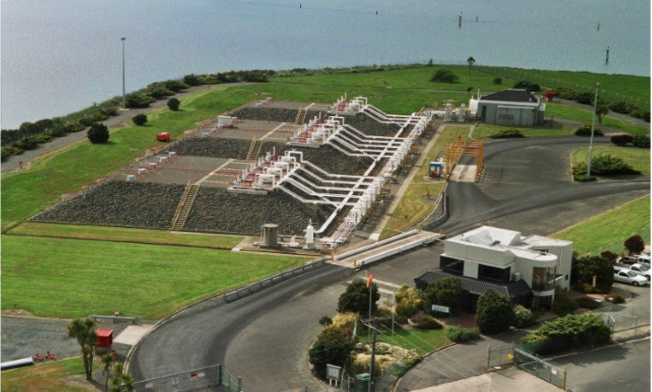
Figure 7 - Gas storage, Port Otago
