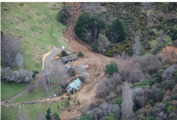
Photo 4: Major Slip affecting properties in Blanket Bay. (From Helicopters Otago BK177, Tuesday, 25 July, 2017)
